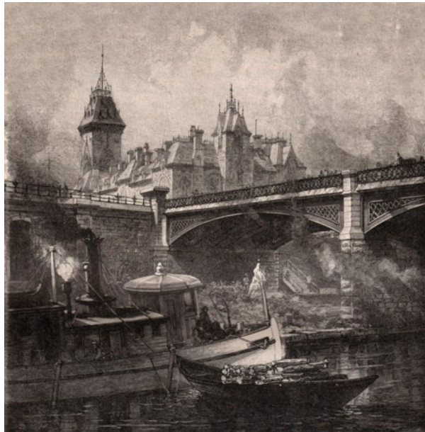
Figure 2.5 Under Dufferin Bridge
